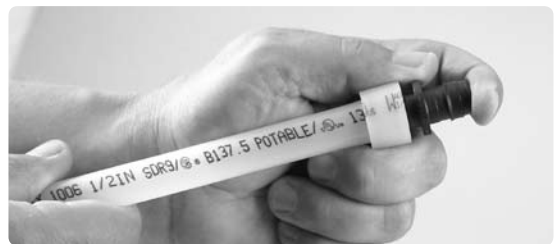
Figure 3-10: Insert Fitting into Tubing
